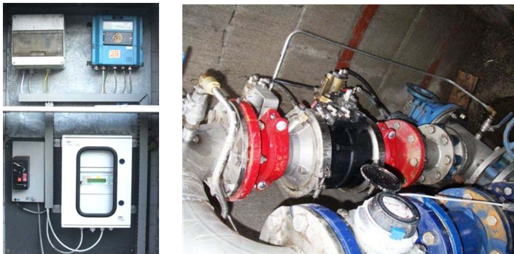
Figure 1.3 Data loggers and building a measurement point
