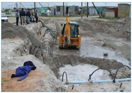
Figure 3. Excavating and De-watering the Site for the 1065 mm Chamber.
