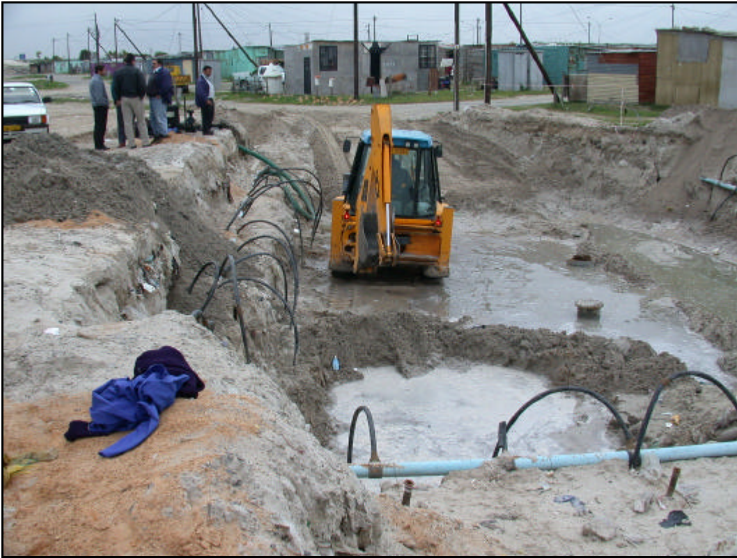
Figure 4: Excavating and De-watering the Site for the 1065 mm Chamber
