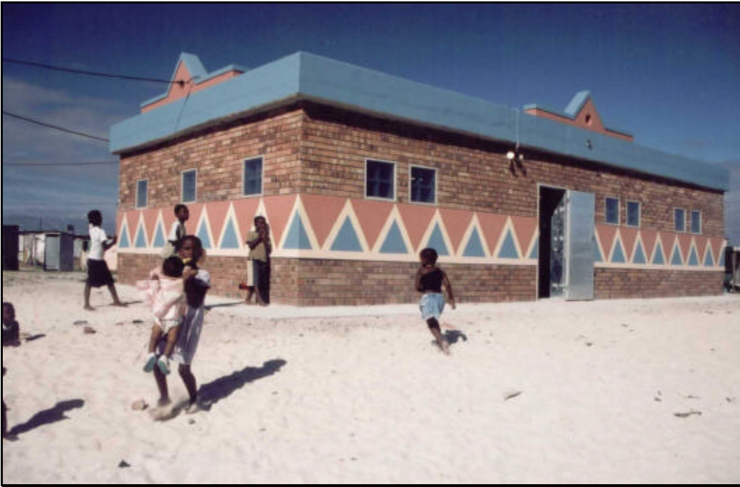
Figure 9: Completed Chamber in Khayelitsha
