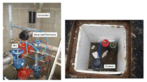
Figure 1.3 Installation of the self learning algorithm system
