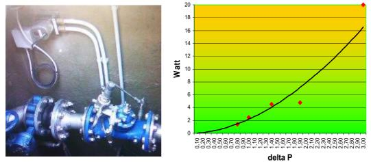
Figure 1.4 Micro turbine and energy produced as a function of delta P.
